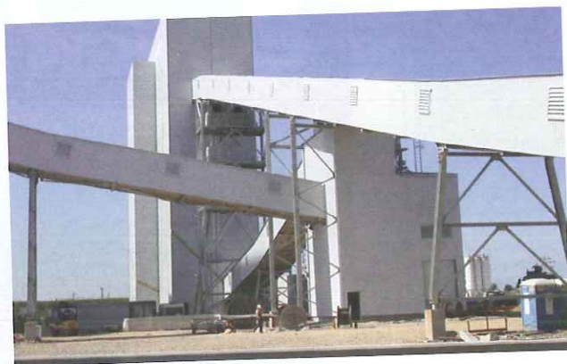
Figure 4. Mill feed bin system.
